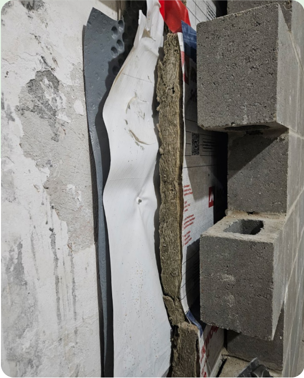
Wall construction prioritizes a tight envelope
