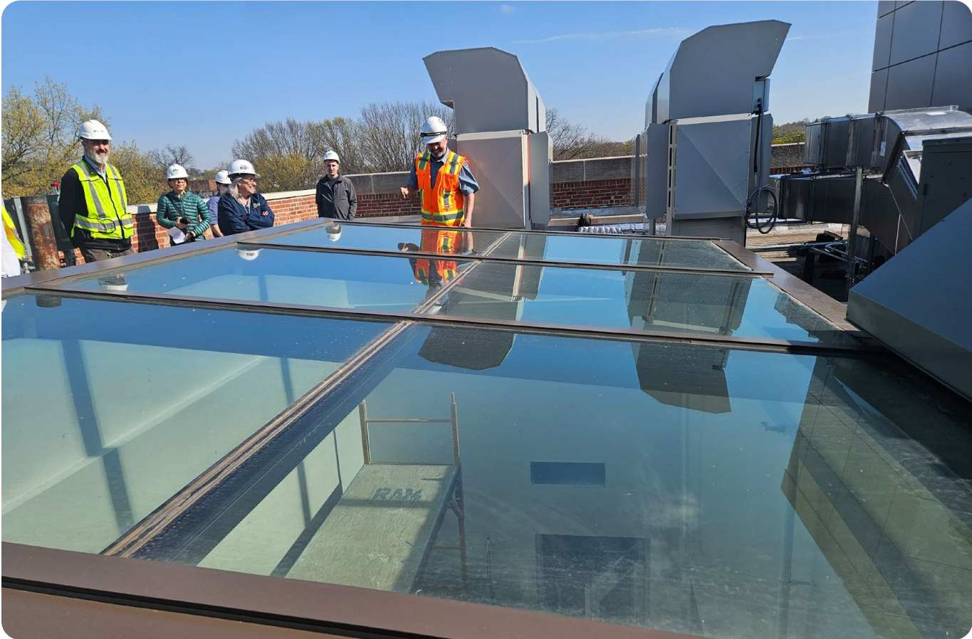
New skylight enhances lighting
