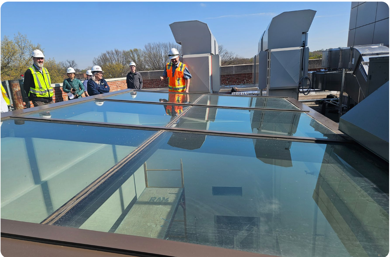
New skylight enhances lighting
